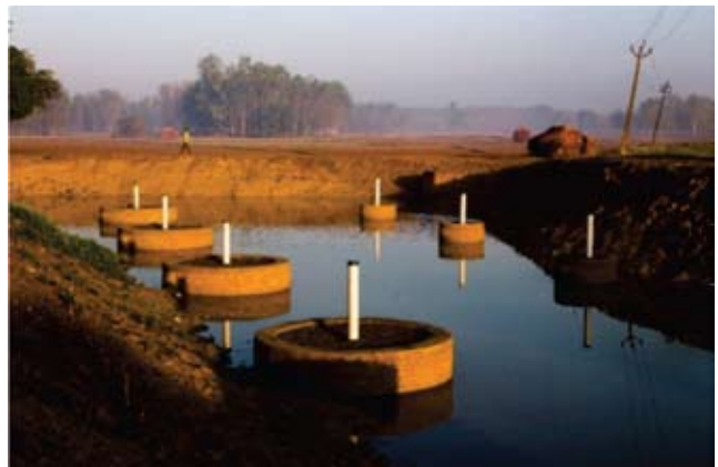
Fig. 6. An unused village pond retrofitted with UTFI technology for flood water recharge in Rampur, Uttar Pradesh
